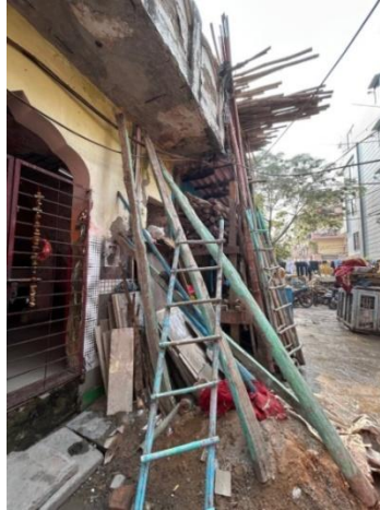
Figure 5: The Temple in Hari Nagar slum Collapsed Due to Heavy Rainfall in August to September 2024
